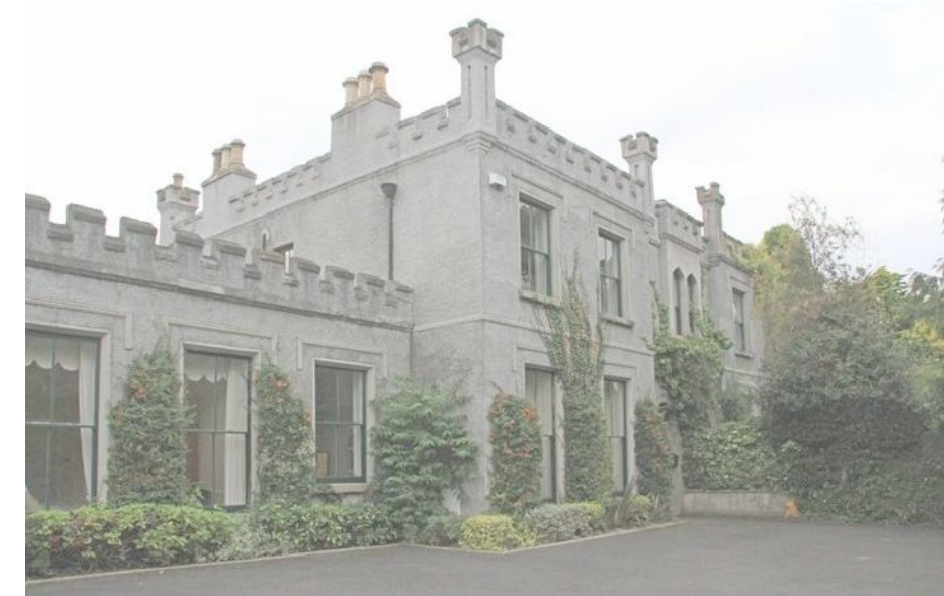
FRANKFORT CASTLE MAIN ENTRANCE SOUTH EAST ELEVATION
